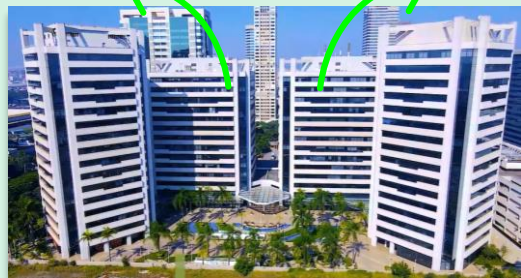
TORRE PADAUIRI (BLOCO B) TORRE DEMINI (BLOCO C)
